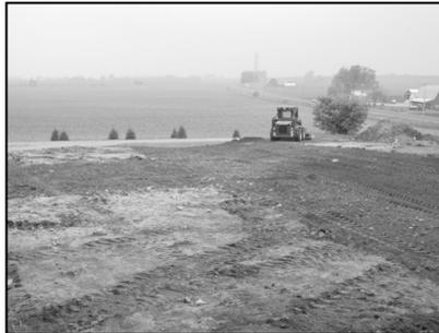
**Setting Grade, Job Site Leveling:** Getting the job site ready is an important step. This is where you set grade, loosen up the material, start obtaining a 2 in. seed bed.
